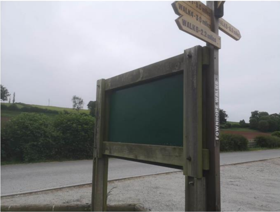
Rear of signage board, available for hosting another cabinet for A2 poster. Plus, fingerpost where the 'Coronation Walk' arrow can be installed
